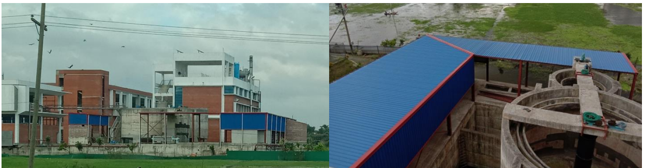
Steel structure project @ Dhaksinkhan
