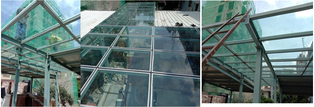
Steel structure project @ Banani Office cum show room.
